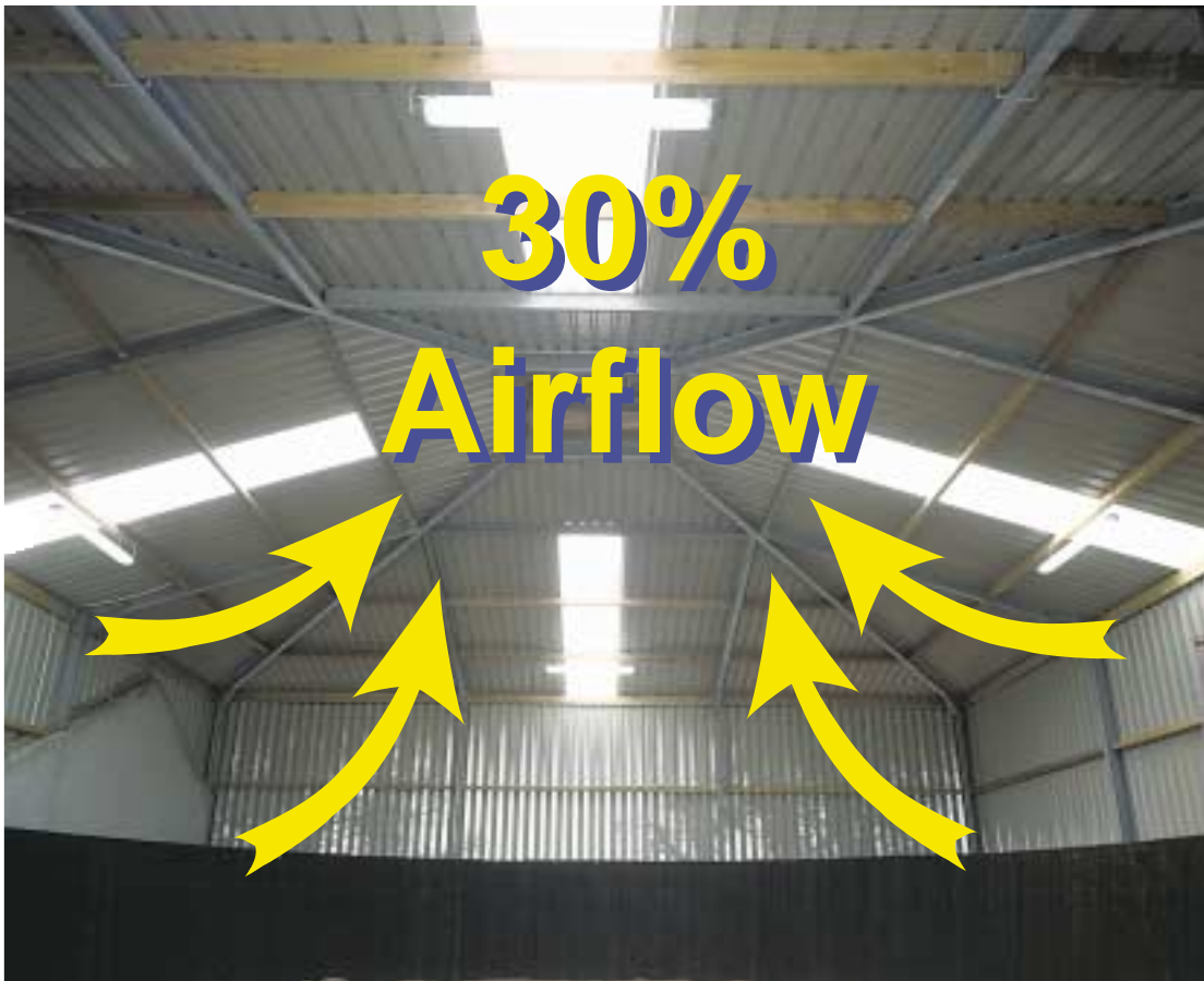
Bottom: Internal view of Equestrian Centre showing Proair® and Profarm® sheet.
